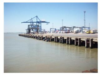
Site: Container Terminal, UK Structure Type: Sheet piled steel piles and tubular piles
